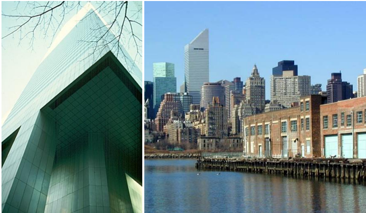
Figure 2 a. The Citicorp building sits 130 feet in the air and is supported by a central concrete core and four perimeter columns, which are positioned at the center of each building face.
