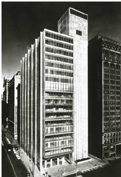
Figure 8. Inland Steel Building
