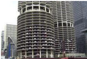
Figure 2. Marina Towers Parking
