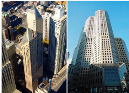
Figure 3. Aerial view of One Mag Mile
