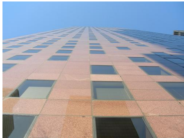
Figure 3. The concrete structure is – unlike the Onterie Centre - clad in rose Granite.
