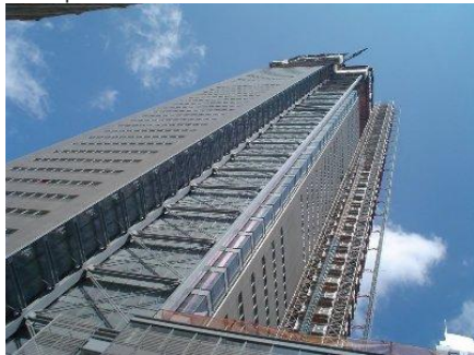
Figure 3. The slender X-bracing in the perimeter notches, orientated in the east-west direction, work in tandem with the braced core to resist lateral loads.
