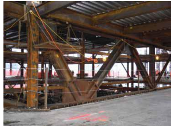
Figure 3. Horizontal truss system employed to transfer additional lateral loads to core
