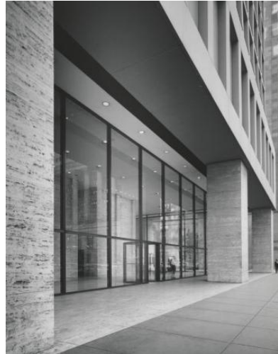
Figure 2. Brunswick Building - at street level
