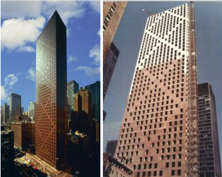
Figure 1.a. The completed 780 3 rd Avenue, NY building showing its 8:1:1 slenderness ratio
