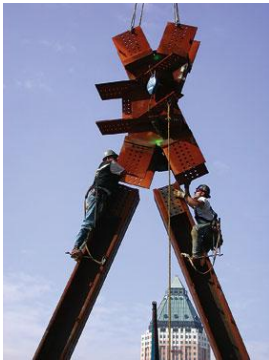
Figure 5. Hearst Tower diagrid under construction.
