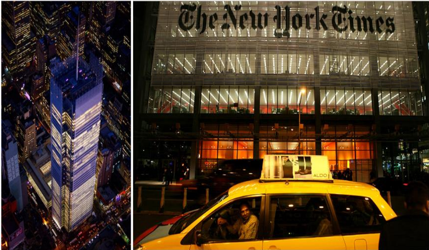
Figure 6 a. The newly completed NYT “green” building has a cruciform plan with exposed steel work. Figure 1 b. A ceramic rod screen, extending far above the roof, blocks out direct sunlight and reduces cooling loads
