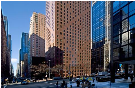
Figure 2. The X form diagonals are formed by infill panels in a stepped pattern. The Plaza with its 22 trees is both elegant and simple in design.
